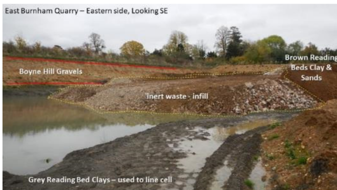
Figure 2 – East Burnham Quarry – showing clay lining and partial infill of the extraction cell.
