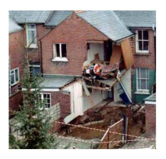
the Reading area as a consequence of subsidence and building development activities. In 1933 only one mine was know but by 2003 over a dozen mines had been recognised. With many have been stabilised by drilling and injecting 'grout'.
