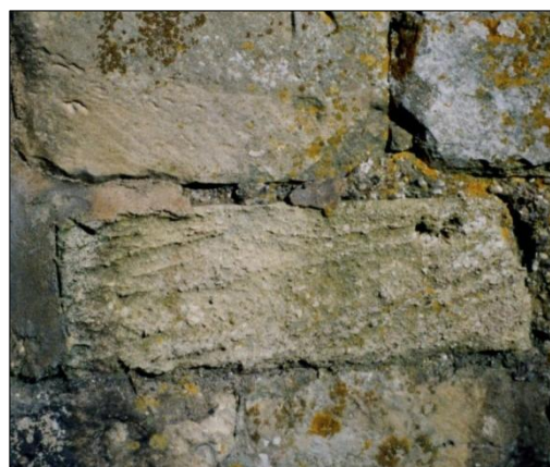
Limestone (Blisworth Limestone) in Thornborough Bridge near Buckingham. The inclined lines are called cross-strata
