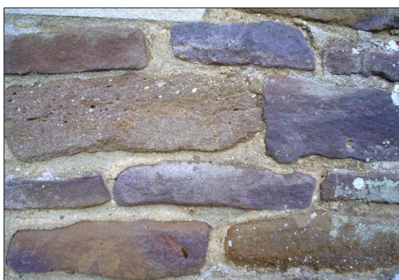
Sandstone (Lower Greensand) in St Mary's Church, Great Brickhill. One block has small pebbles scattered in it. The dark colour is an iron oxide cement.
